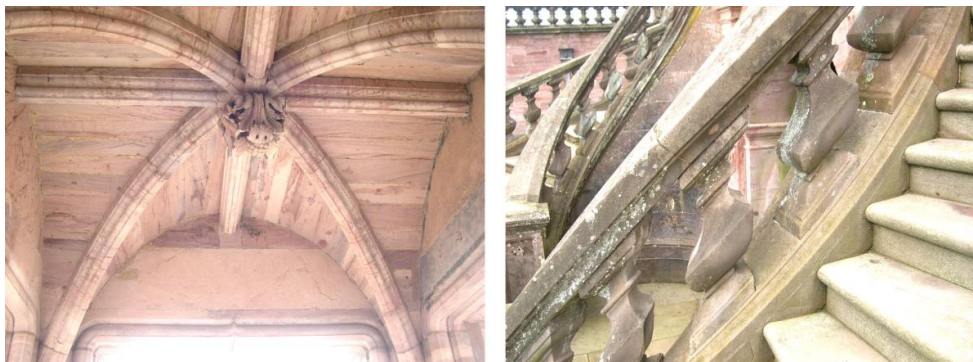
Figure 7: Vault above main entrance and balusters of stair
