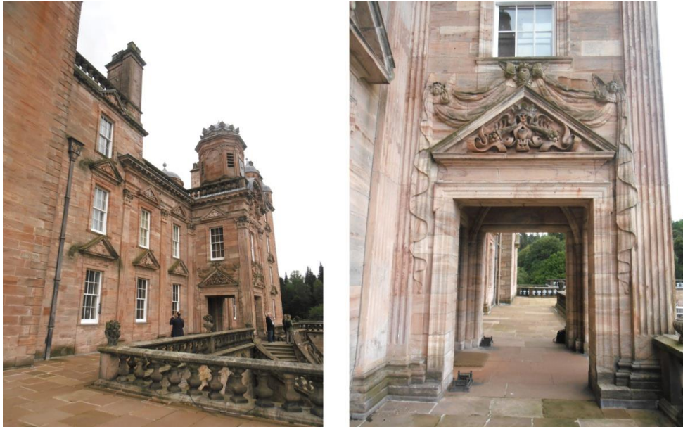
Figure 6: Front terrace and stonework at the main entrance
