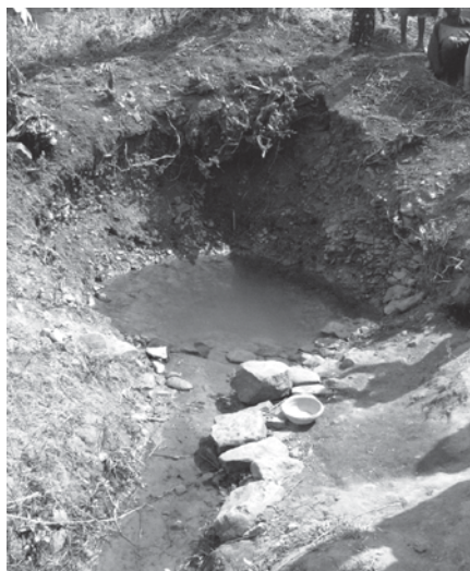
Figure 1: Unprotected spring in a field in Village A. This source is used for all purposes, including drinking.
