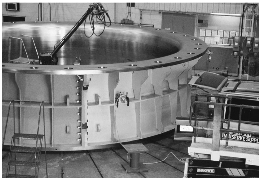
Fig. 4 Hydropower wicket gate bearing ring during VSR treatment. Material – cast steel, with welded repair. The ring has an internal diameter of 5.6 m. Approximate weight is 40 tonnes. Photograph courtesy of the VSR Group of Airmatic Inc
