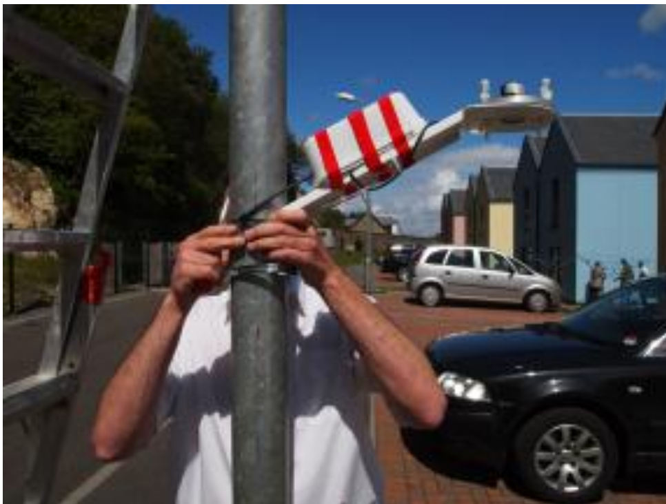
Figure 6.21 – Pyranometer Installation
