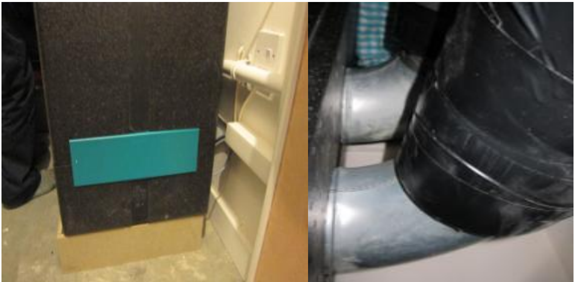
Figure 6.22 – PassiveHouse MVHR Ducting Unit; insulation issue
