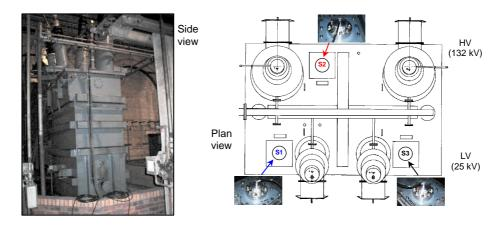
Figure 11: An 18 MVA Single Phase Traction Transformer Equipped for UHF Monitoring
