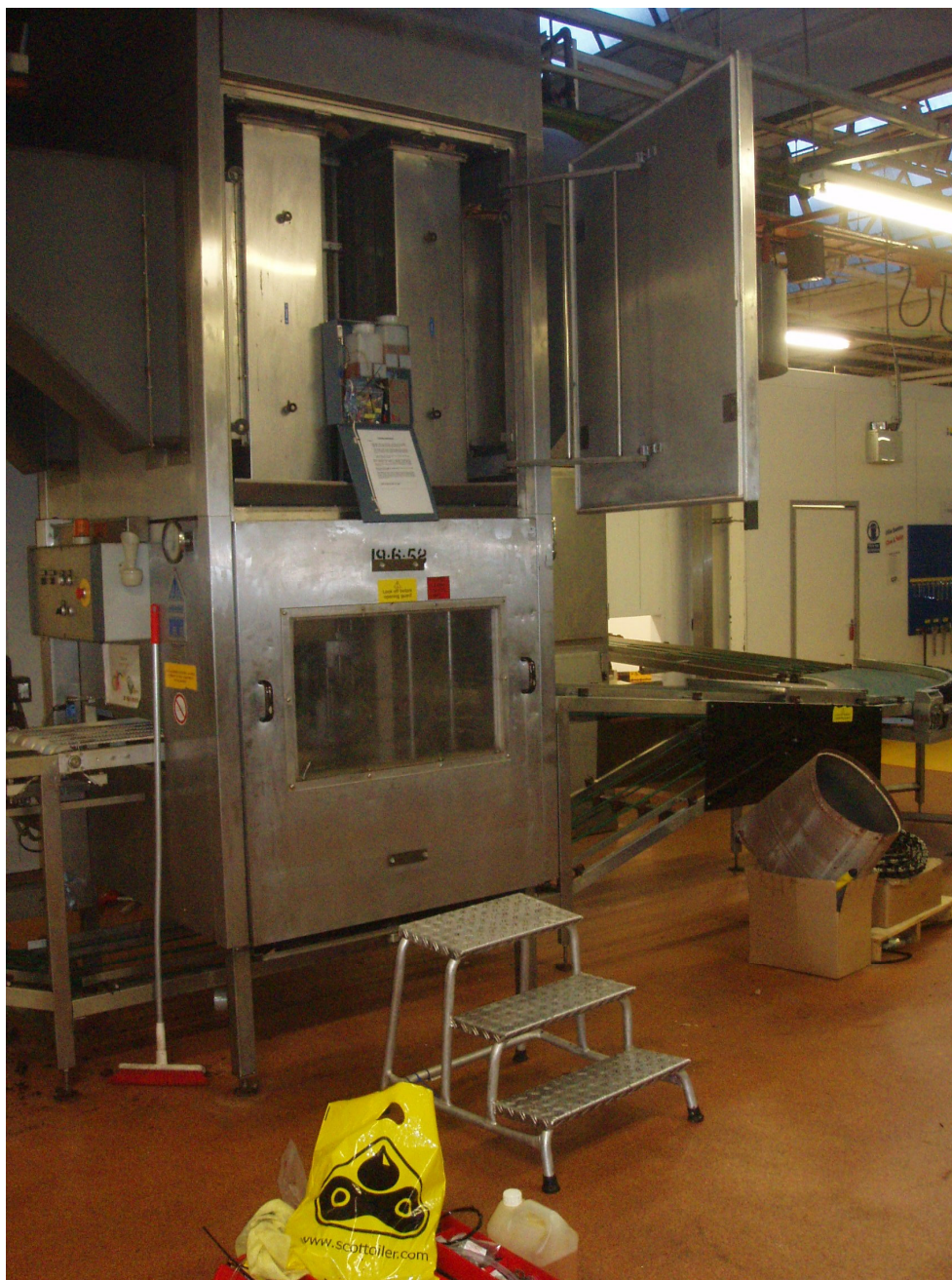
Prototype I Installation
