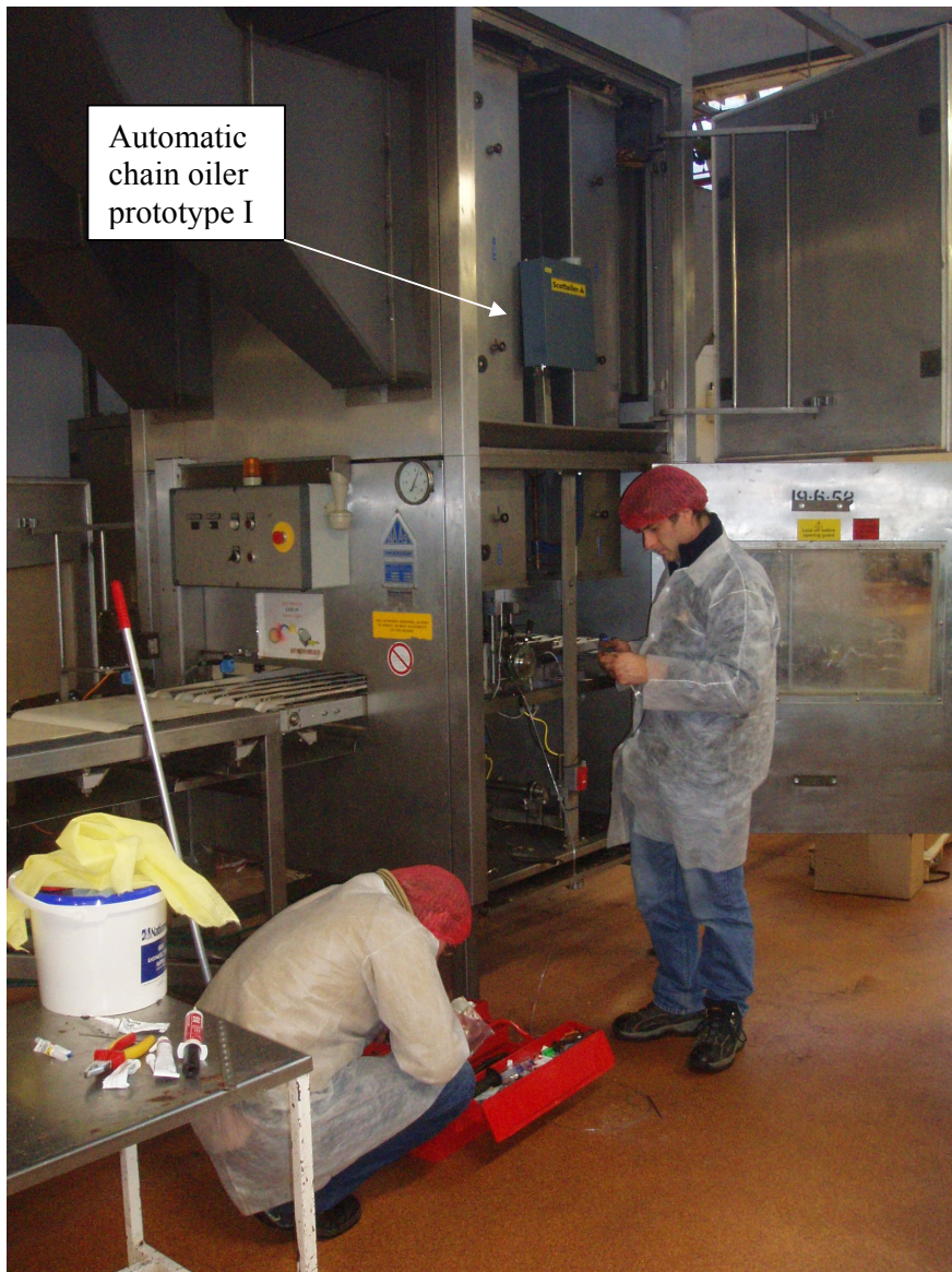
Figure 6-10 Installation of the first oiler prototype inside the cooling tower.
