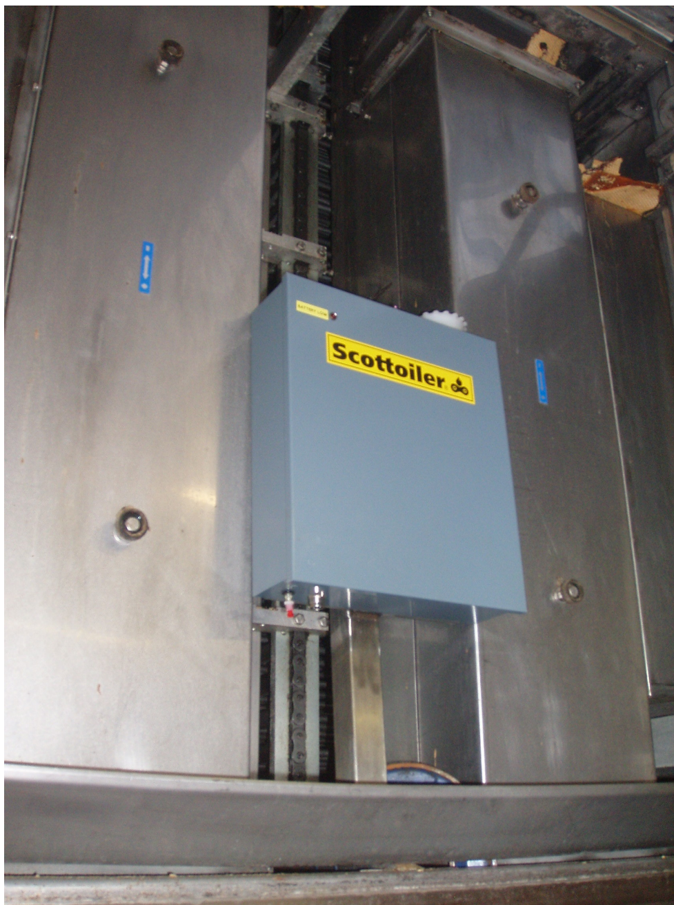
Prototype I Installation
