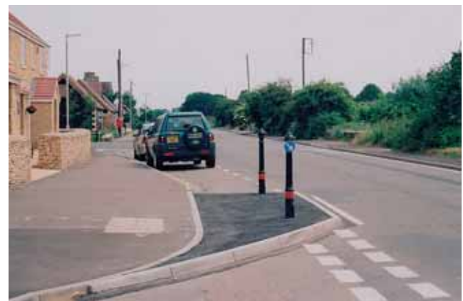
(d) Build-out at junction with Collett Place
