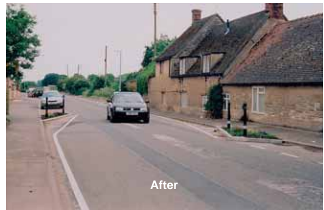
(b) Build-outs with planting north of the junction with Collett Place (looking south)
