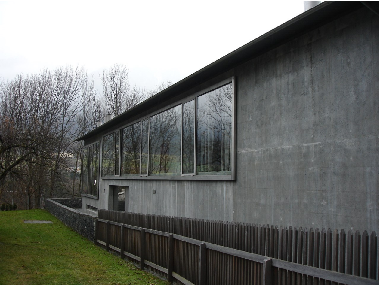
Figure 9 Window frames hang picture frame-like similar to those used in..
