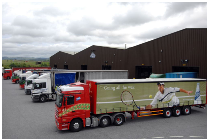
Figure 7: Exterior of Highland Spring Warehouse and loading area
