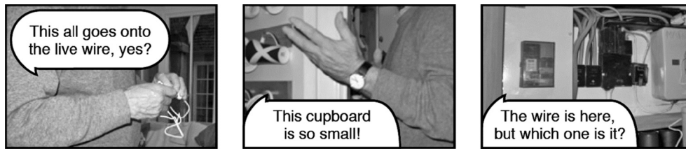
Fig. 5. A very common challenge was ease of access to the electricity meter and identifying the correct cable to clamp the sensor onto.
