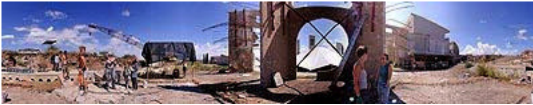
Arcosanti: East Crescent under construction, 1999
