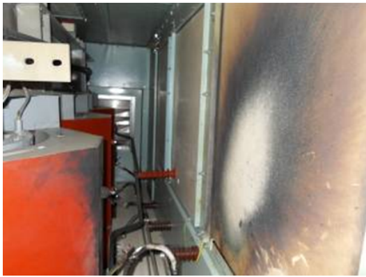
(a) Evidence of vaporised conductor due to an arcing fault on a marine vessel transformer [Daf09]
