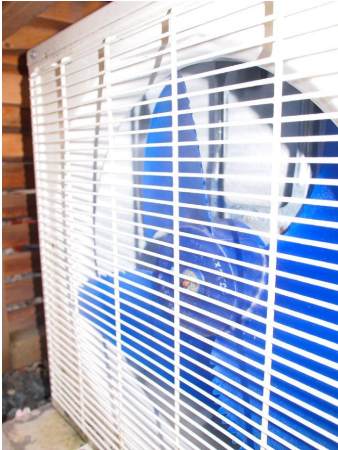
Figure 4 - Frost build up on ASHP. Image taken at 5°C in Dunoon, Scotland
